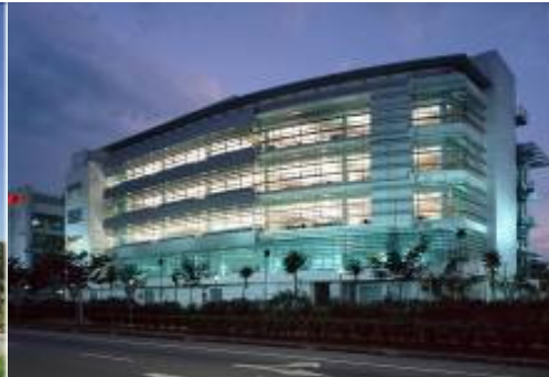
Quill Building 4 – DHL 2
