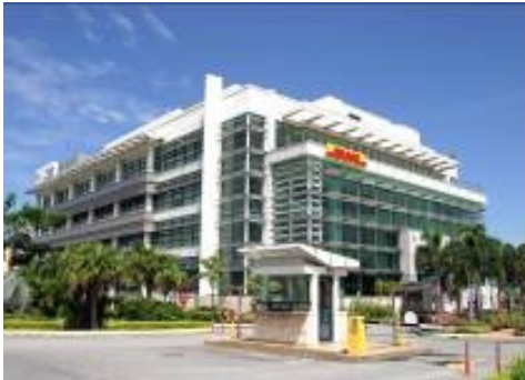
Quill Building 1 – DHL 1
