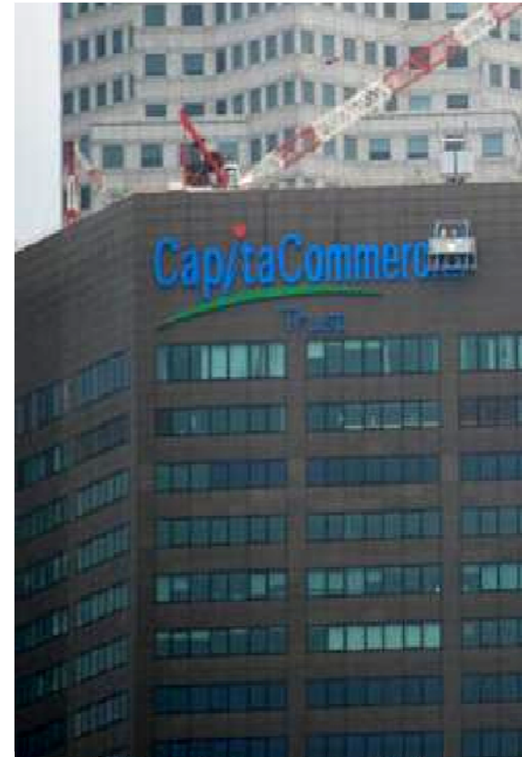
Installation of logo on building
