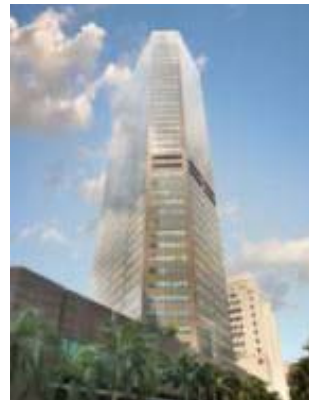
Six Battery Road
